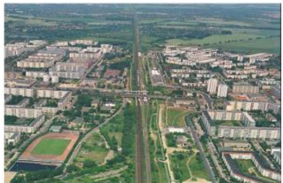
'Complex residential construction', East Germany 1970s – 1980s
